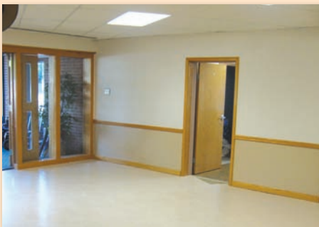
The remodel of the front entrance of the Metro facility.
