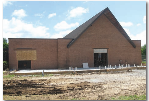
Construction began in May 2013 at the Fairview Heights Metro Facility.
