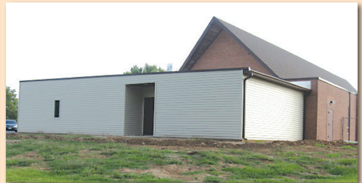
The 1,500 square foot addition began close to completion.
